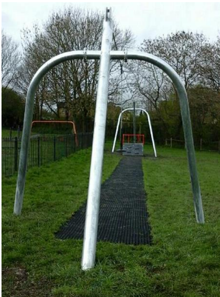
Picture two: Example of metal framed ariel wire with rubber matting and landing platform.
